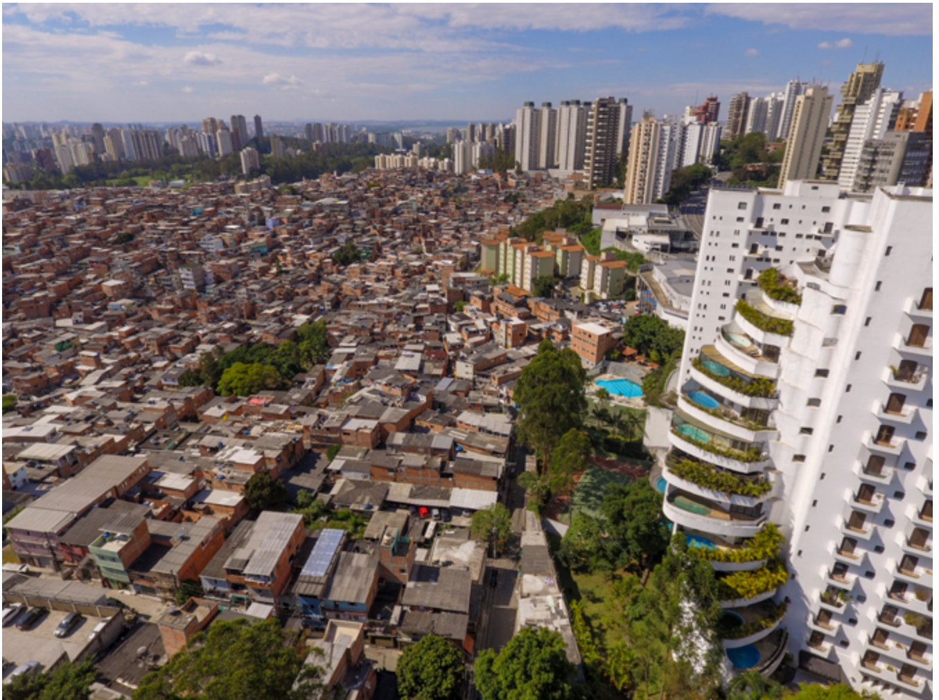
Figure 10 – Contrast in neighboring areas in housing conditions
